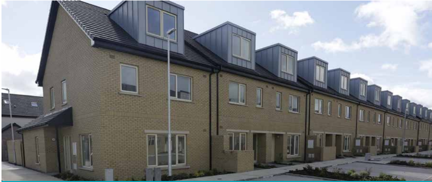
Pictured, 52 new Part V social homes at the Parklands development in Citywest, Dublin, funded by Dubco Ireland through the CU AHB Fund.
